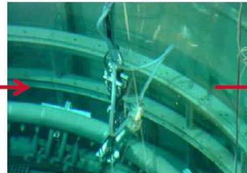
Cutting of core spray tube
