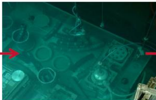
Post segmentation of core spray tube
