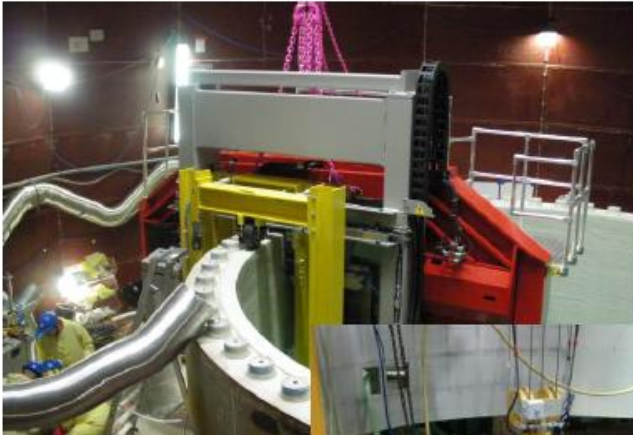
Vertical segmentation of RPV flange
