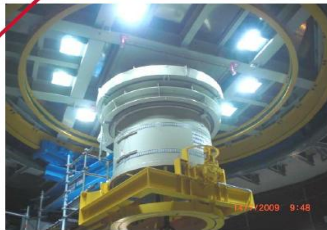
5,5t lifting unit
