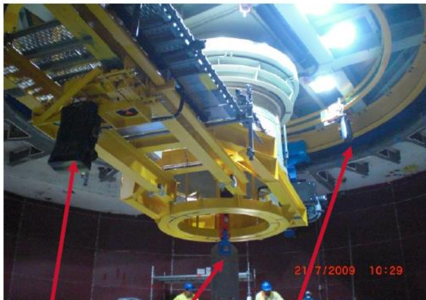
2t lifting unit
