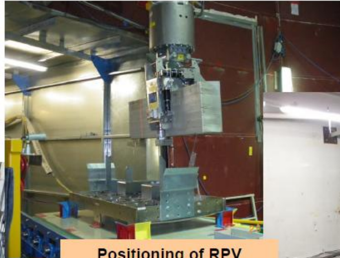
Positioning of RPV segment for transport to container loading station
