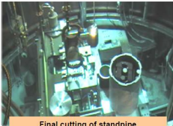
Final cutting of standpipe
