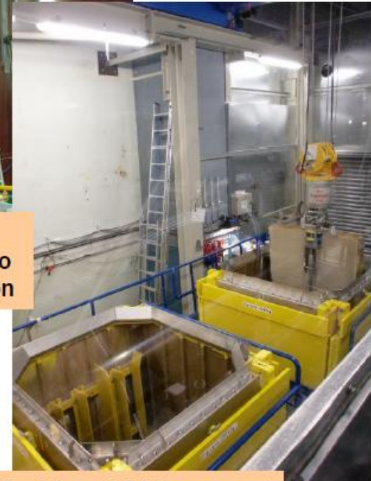
Packing of RPV segment into KONRAD container
